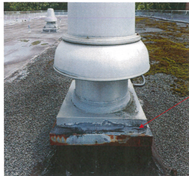
Photograph 19: Gray Exhaust Vent Caulking
