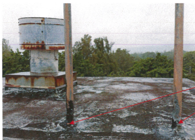
Photograph 1: Roof, Black Sealant around Metal Handrail
